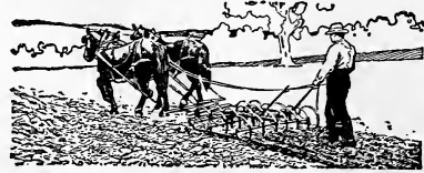
HARROW, McCORMICK-DEERING, SPRING TOOTH, WITH LEVERS
